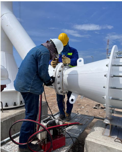
Flame arrestor vent stack- HOCOL 2023
