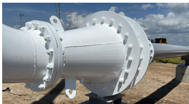
Flame arrestor vent stack- HOCOL 2023
